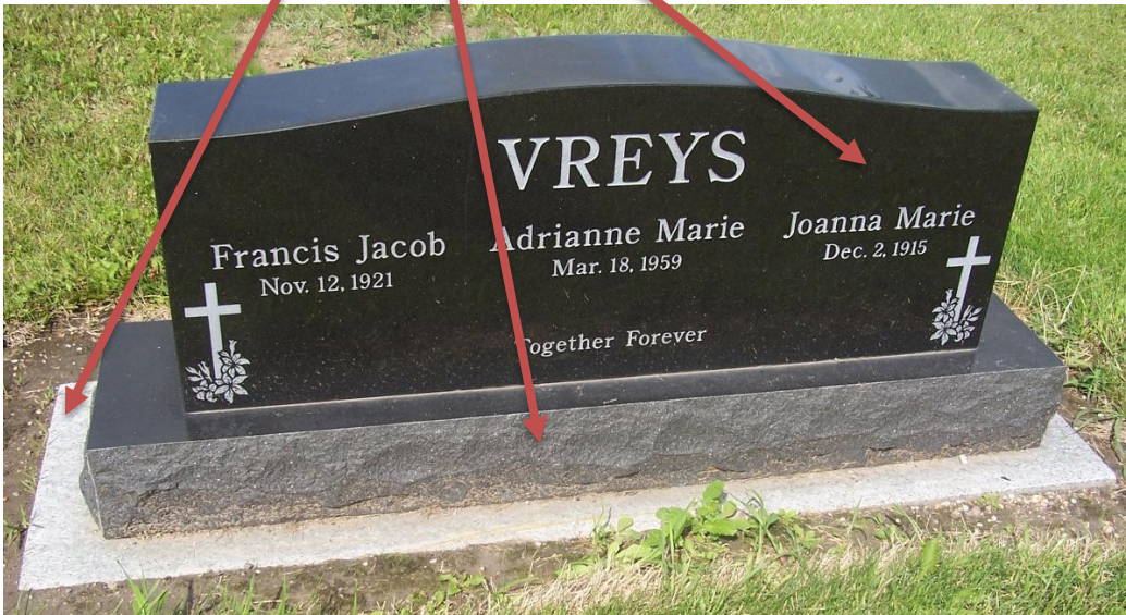
Upright Monument: Foundation, Base and Monument
